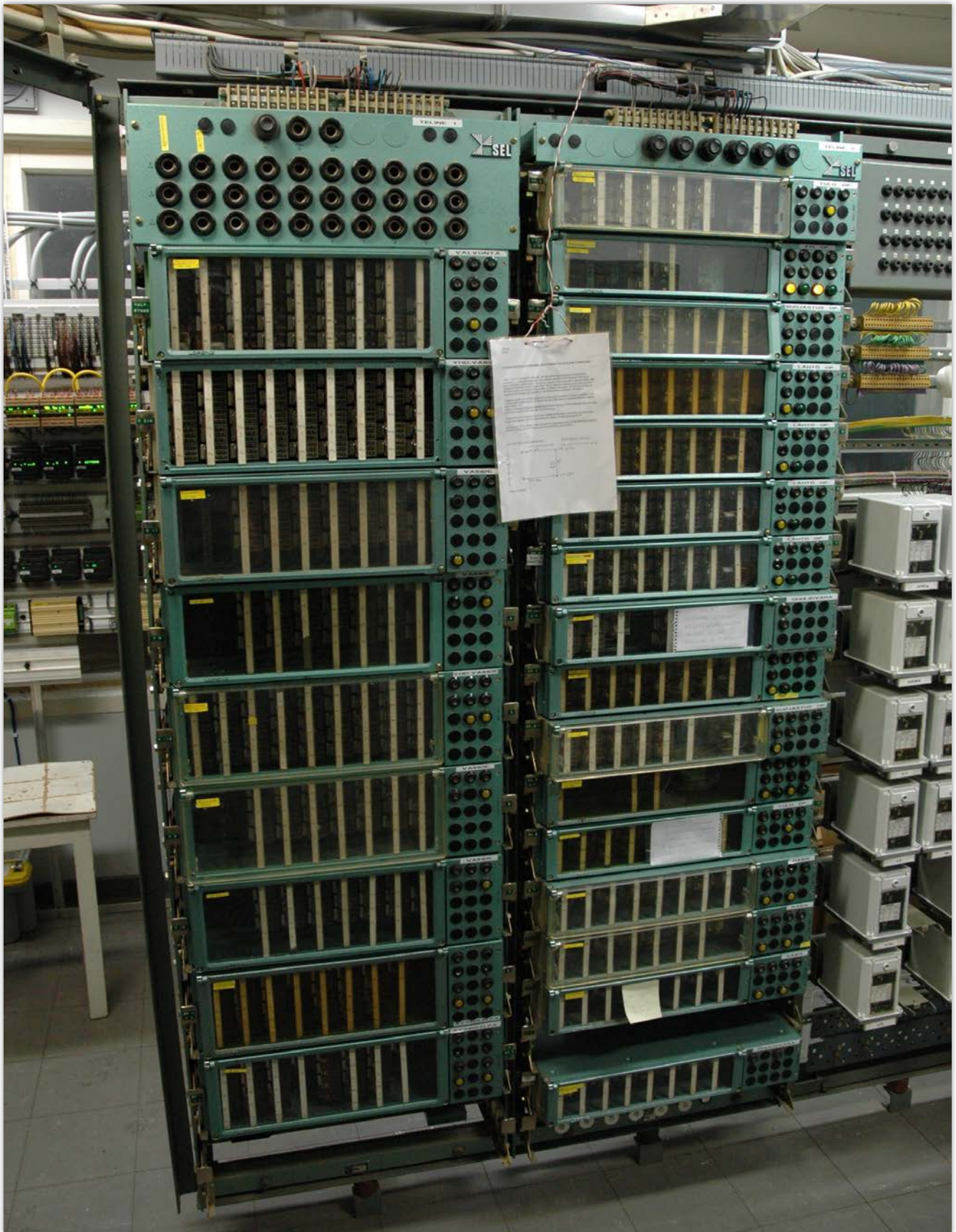
Figure 86: Relay groups of design SpDr L 60
