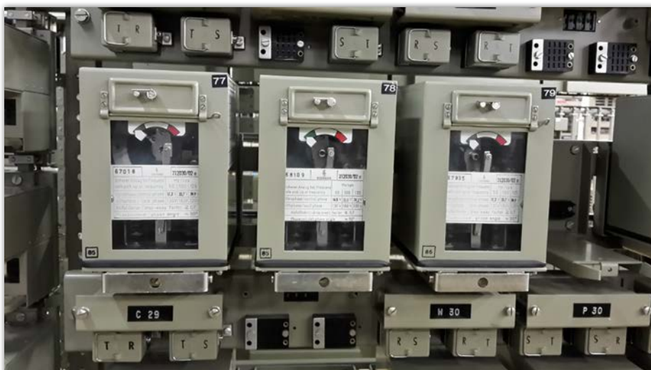
Figure 80: Two-layer motor relays in an SpDr S60
