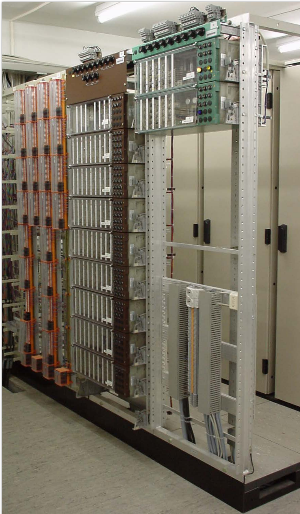
Figure 88: Relay groups in an electronic interlocking of type ESTW IL 90
