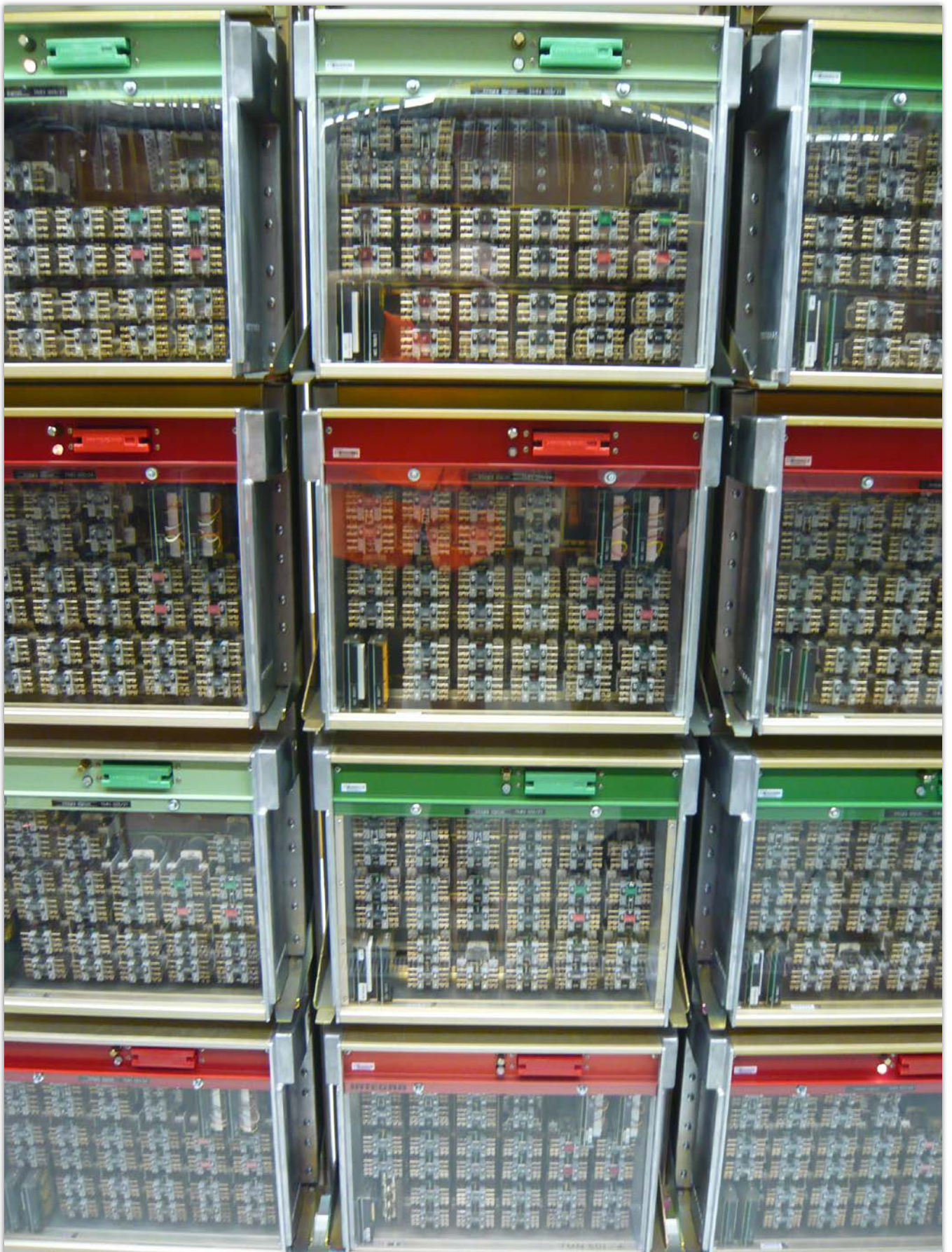
Figure 87: Relay groups of design Do 67
