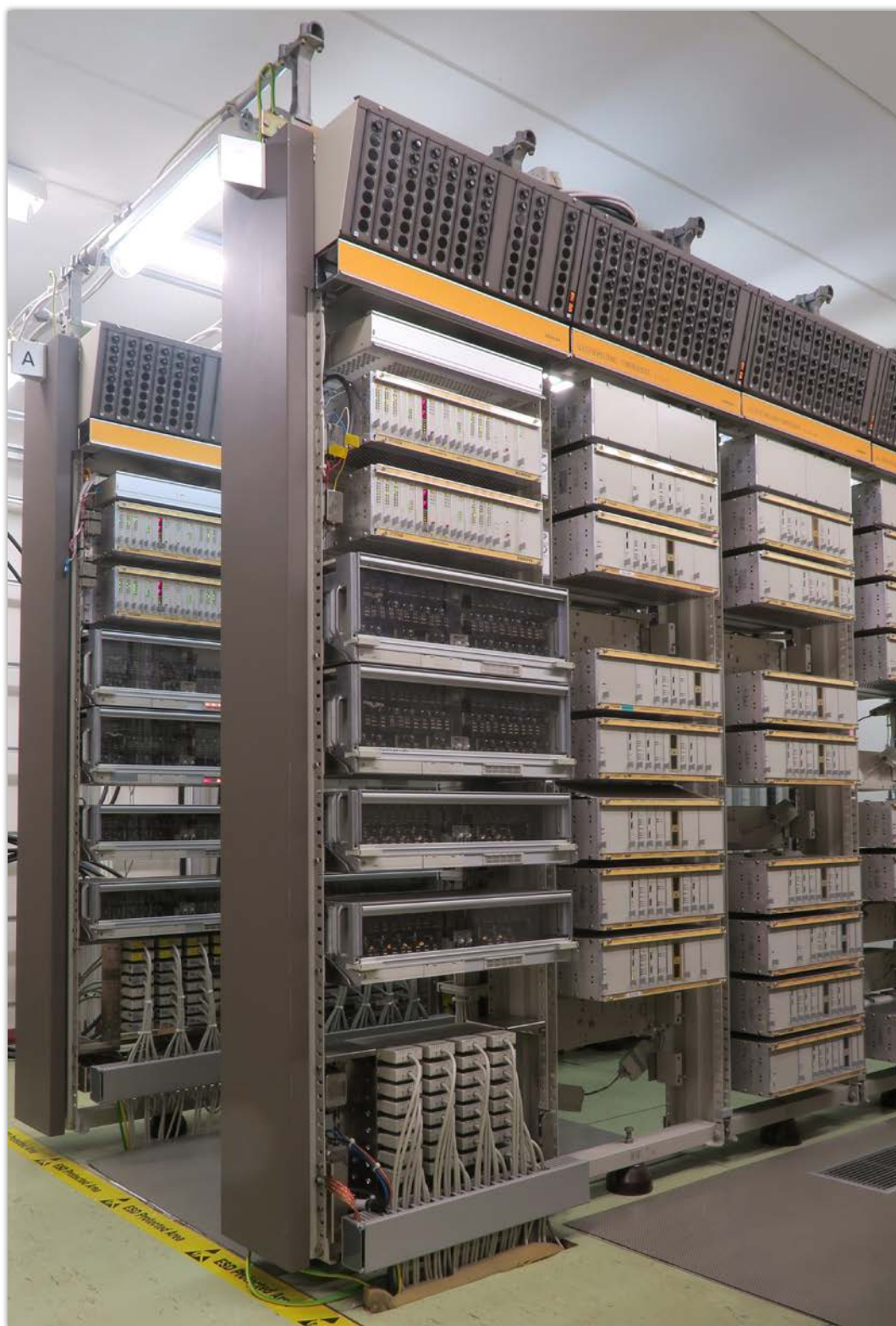
Figure 90: Relay groups in an electronic interlocking of type SIMIS-C
