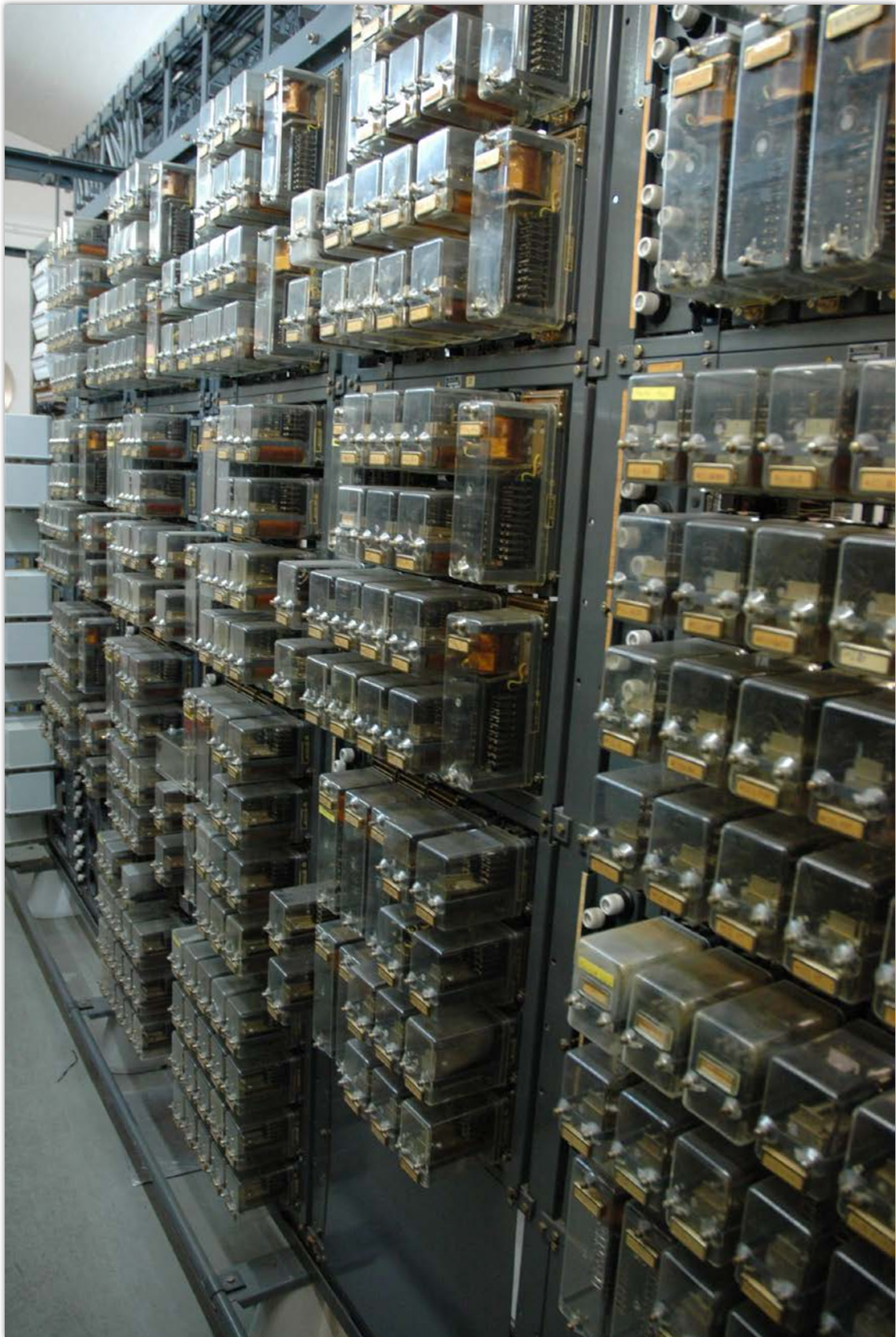
Figure 83: Relay groups of design WSSB II
