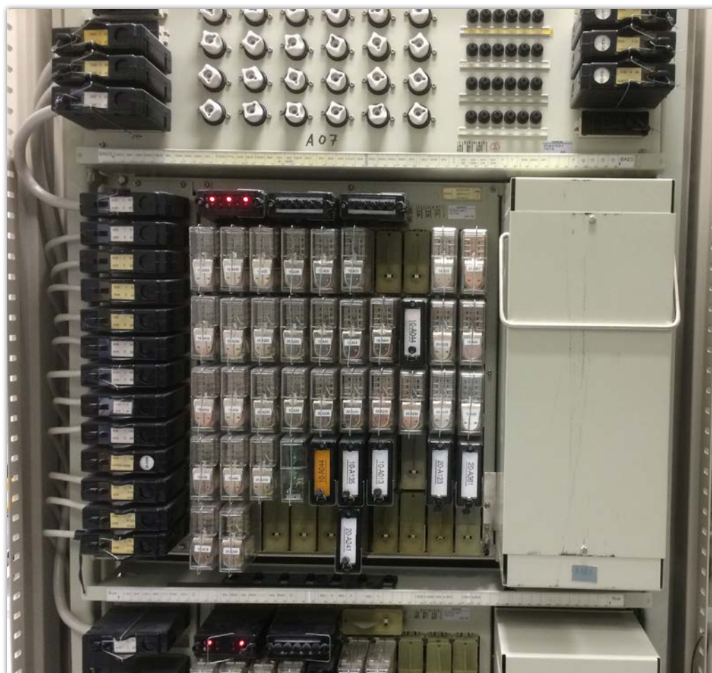
Figure 84: Relay group of design WSSB III
