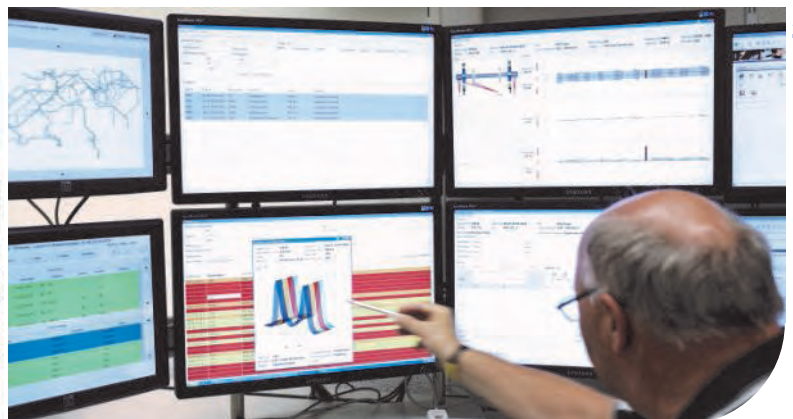
Figure 2: Intervention Centre workstation in Erstfeld
